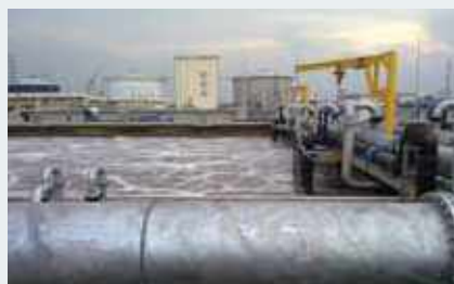
Wastewater treatment, Hanoi, Vietnam The wastewater treatment plant, Yen So Park, treats 50 % of Hanoi's wastewater. More than 90 VSDs are installed, of which 12 450 kW VLT® AQUA Drives control the blowers.
